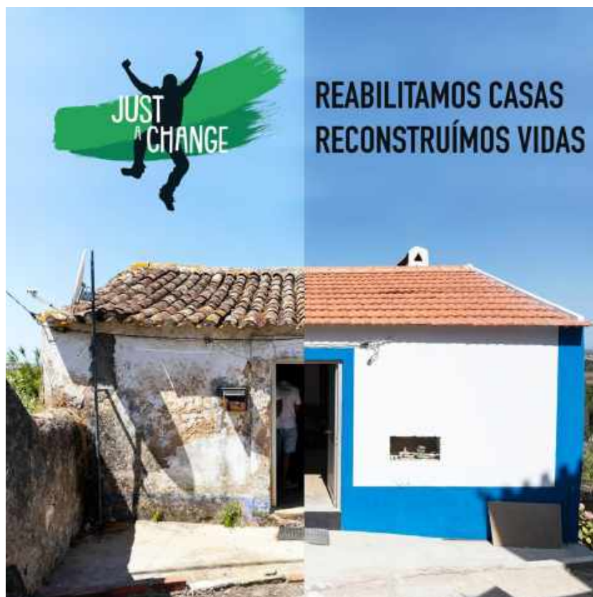
Figure 16 Typical before and after full intervention
