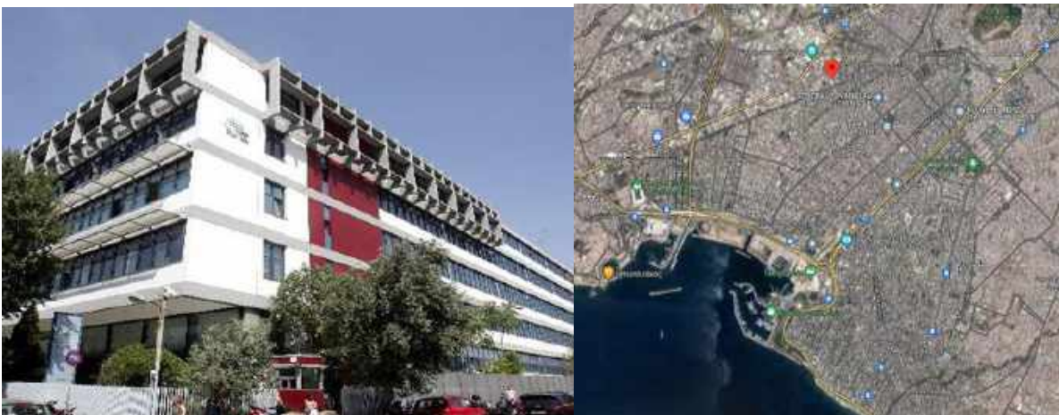
Figure 17 Offices for Demo 5
