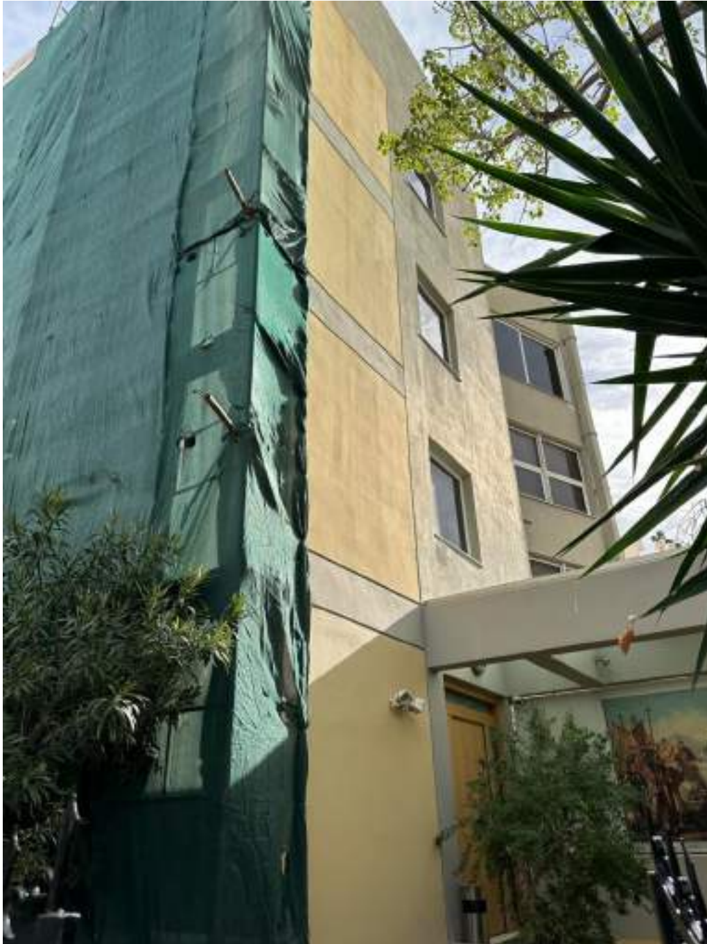
Figure 3 Museum Facade during and after the renovation
