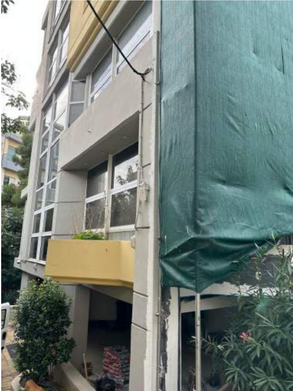
Figure 2 Museum Facade during and after the renovation 1.
