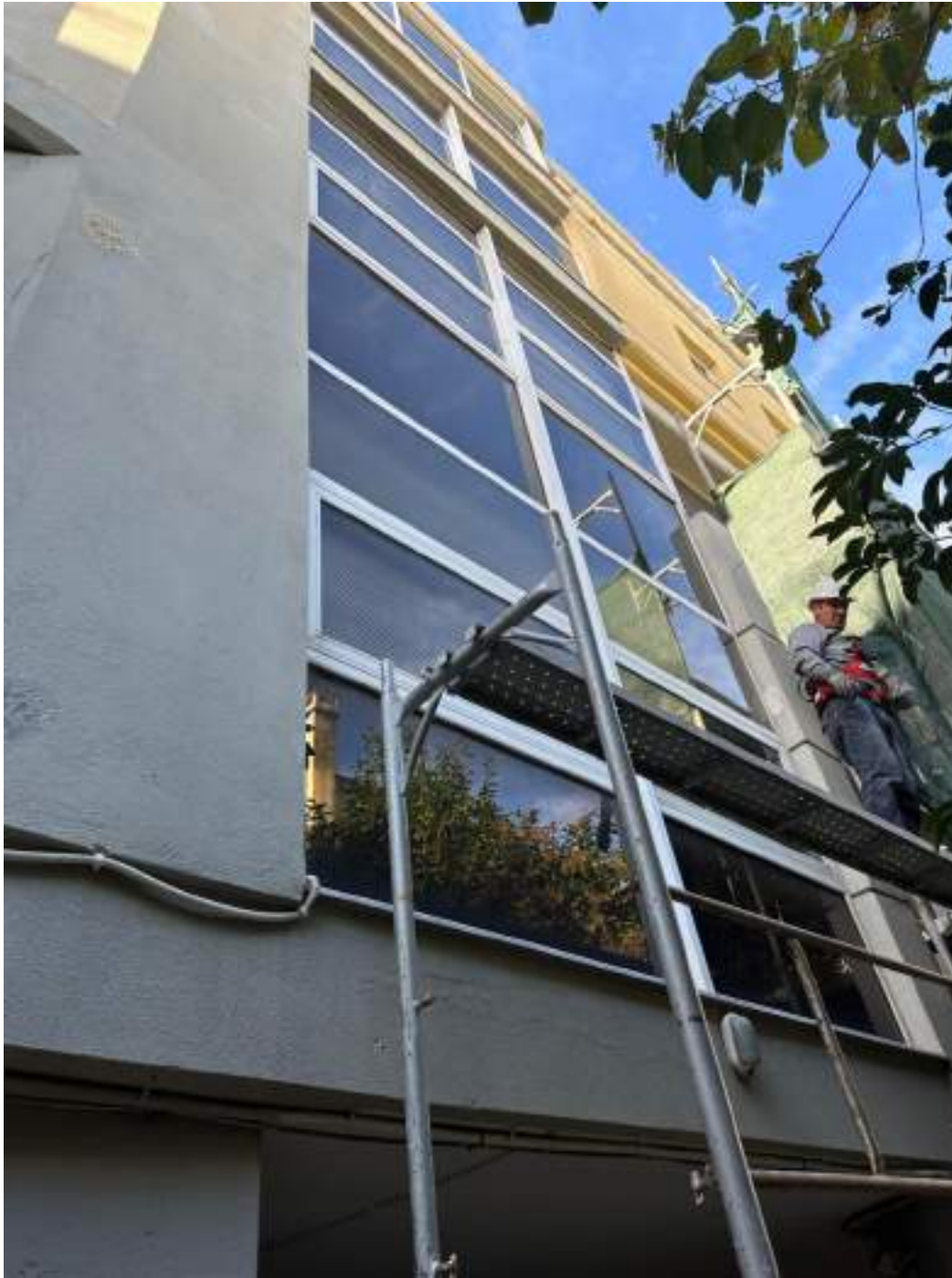
Figure 4 Museum Facade during and after the renovation
