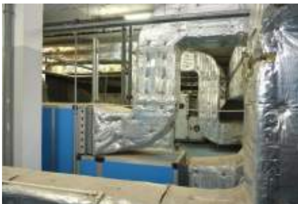
Figure 21 Existing air handling unit (AHU)
