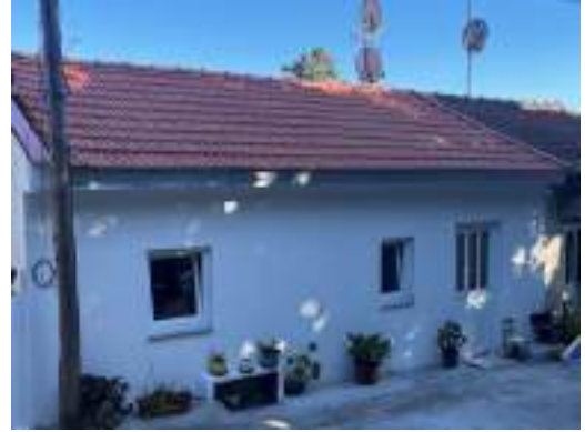
Figure 11 House n. 1 - Porto after
